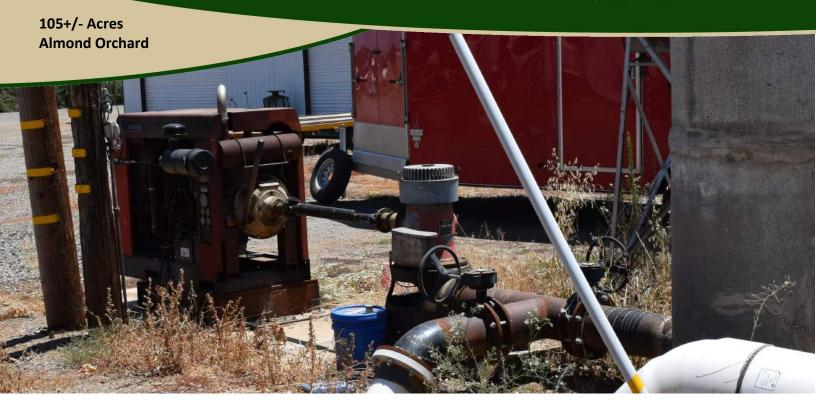
The 80 Hp Ag well is currently being driven by a diesel motor. This is for use in drought situations only. The orchard is primarily irrigated with Orland-Artois Irrigation water.
