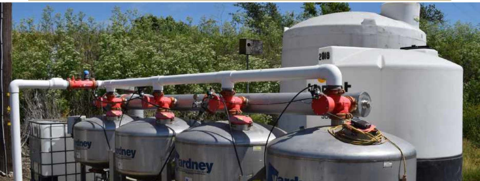
Sand media filters & fertilizer tanks at the pump station on the farm
