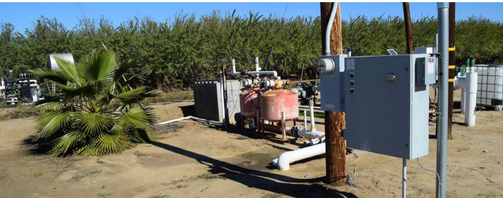
Lift Station & Sand-Media Filters
