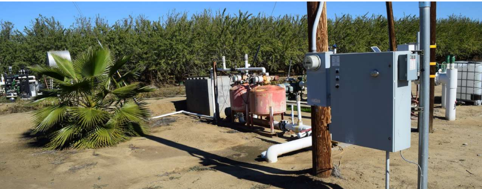
Lift Station & Sand-Media Filters
