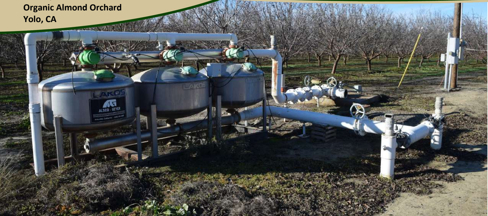
Submersible Pump & Sand Media Filters
