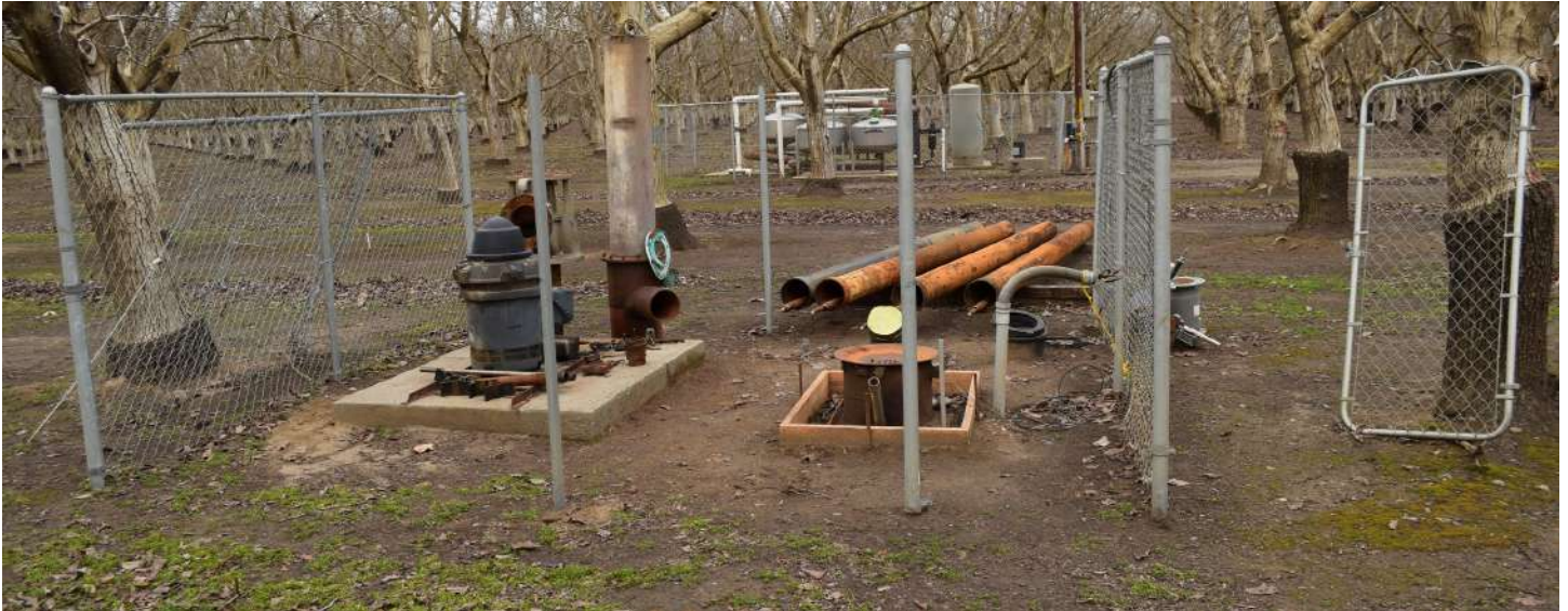
Filter Station & Submersible Well That Serves As A Fill Station
