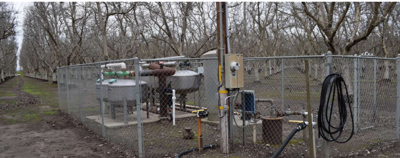
Filter Station & Submersible Well That Serves As A Fill Station
