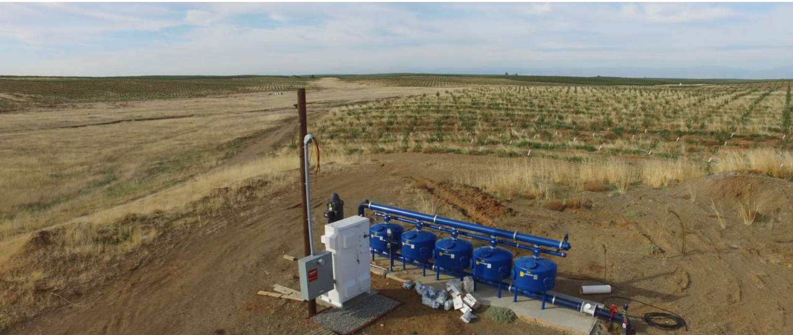
Well#2 With Filters & VFD
