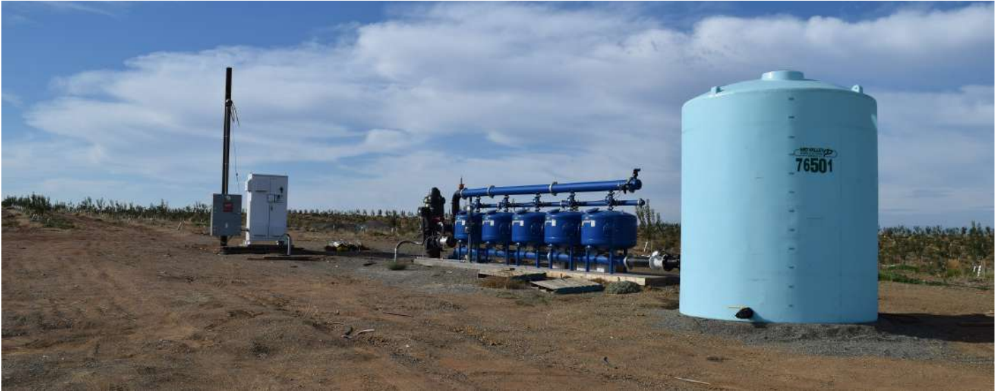
Well#2 With Filters & VFD
