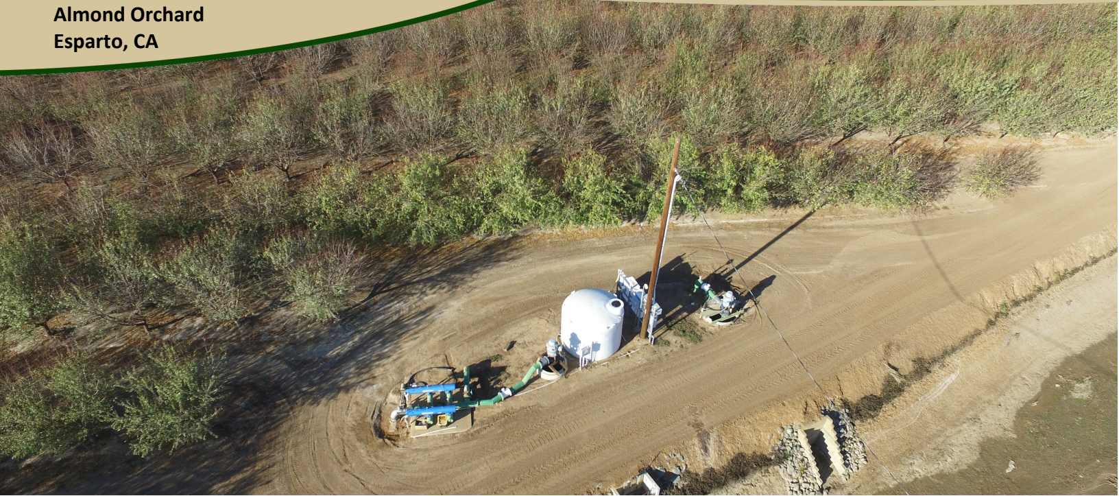
Water District Canal, Lift Pump, Fertilizer Tank
