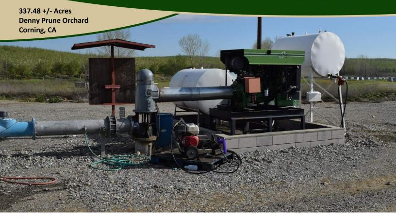
John Deere Diesel motor at one of the well sites. 1st class setup includes filter and fertilizer injection
