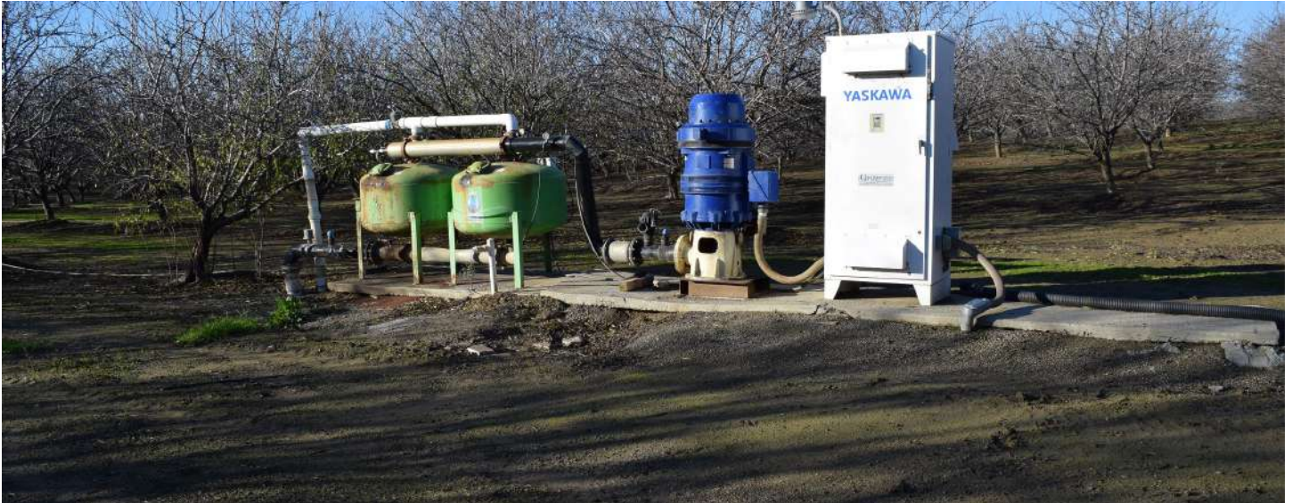
Irrigation Well with Sandmedia Filters and VFD
