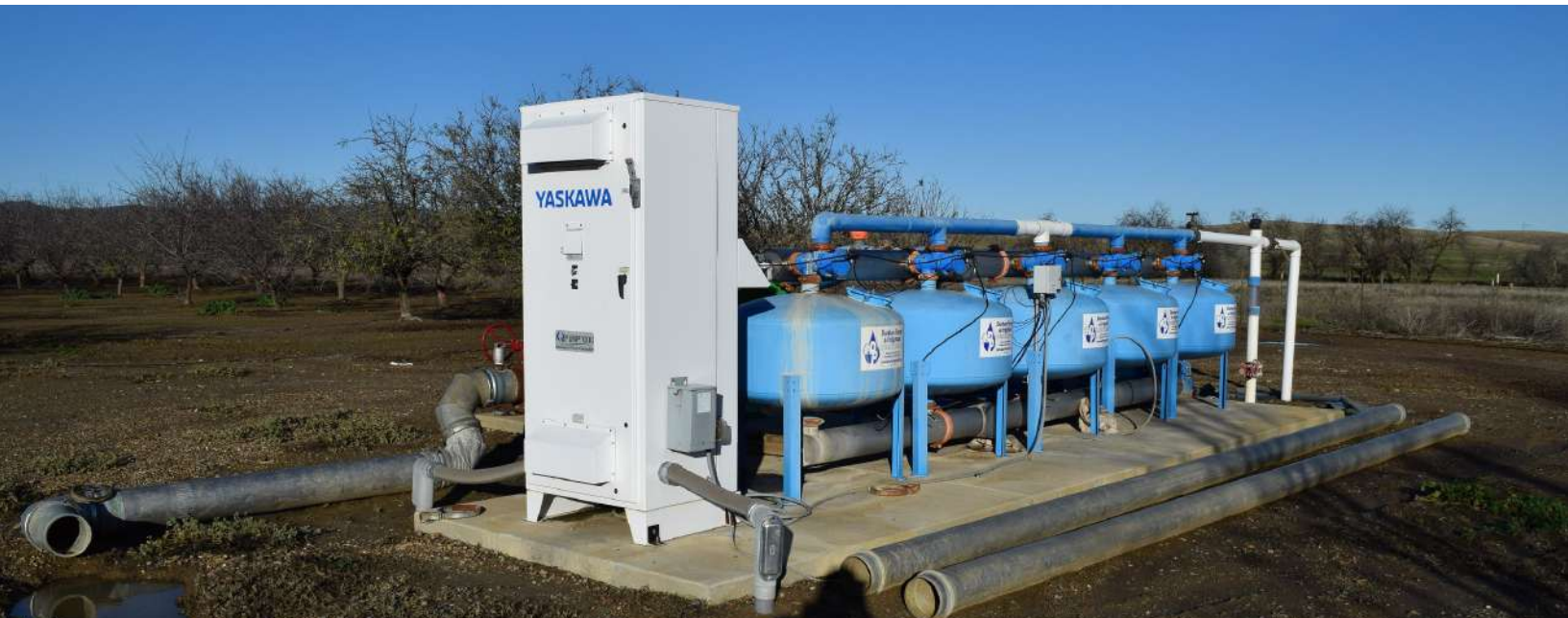
Irrigation Well with Sandmedia Filters and VFD
