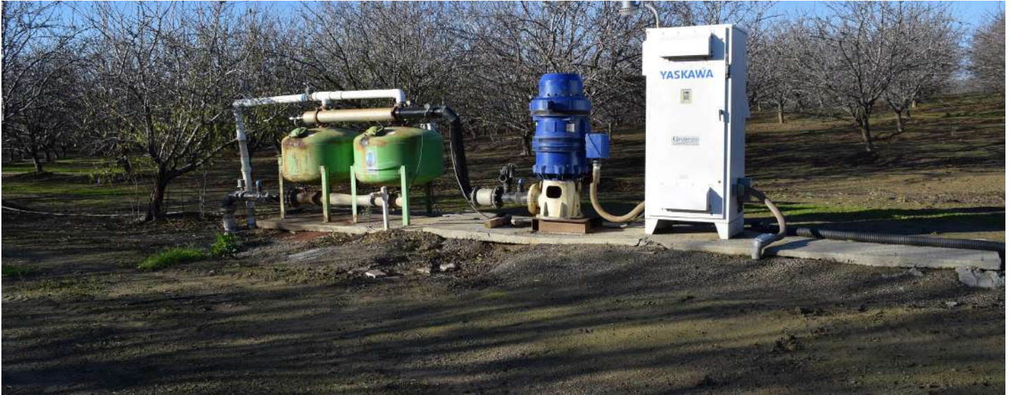
Irrigation Well with Sandmedia Filters and VFD
