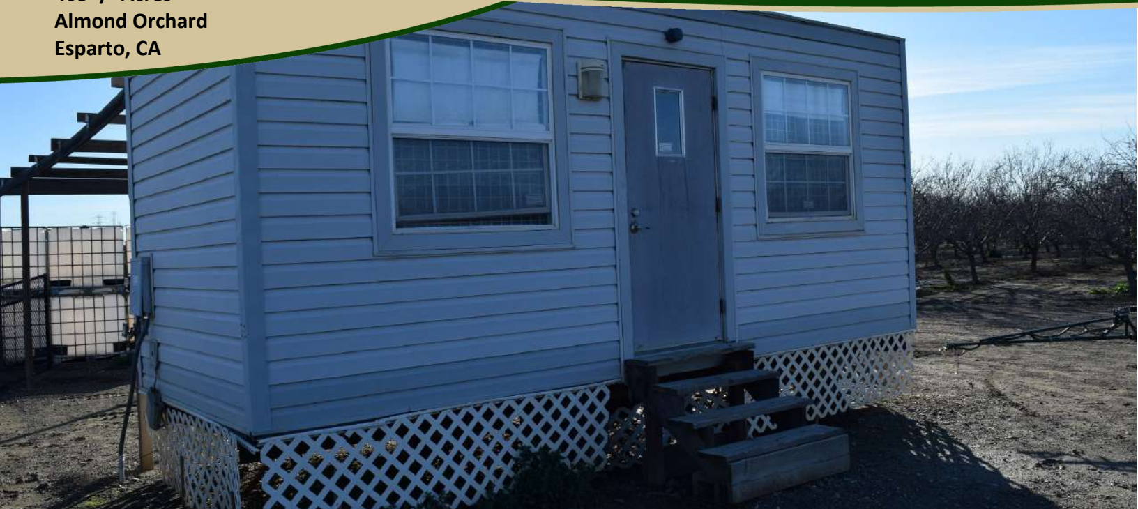
Farm Office and Equipment Yard
