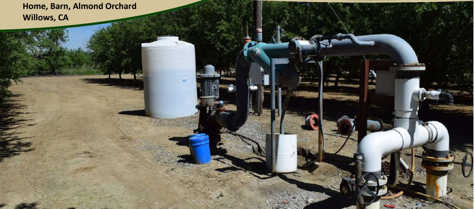
Agricultural Well, Filter, and Acid Tank
